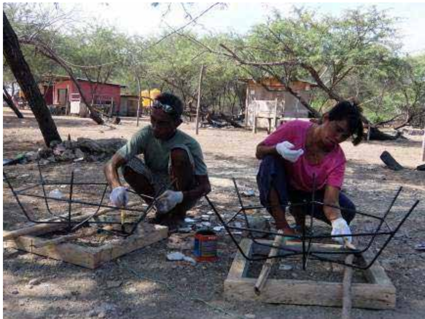
Figure 11. Simple and effective spider frame structure for coral rehabilitation. Man and woman can participate in the process using locally sourced materials.
