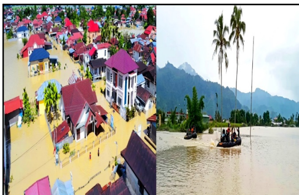
Extreme rain fall that occurred in 2023 in Kerinci Regency, Jambi caused a flood disaster that damaged agricultural land, public service facilities and people's home
