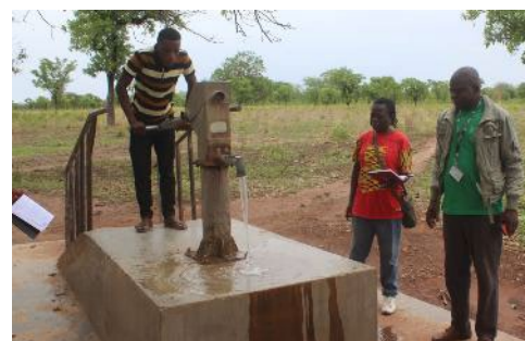
Image 8. Borehole in Mognegu I, repaired using VSLA funds
