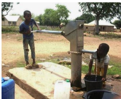
Image 4. Functioning Borehole in Kiape, Savannah Region
