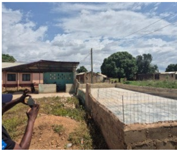
Expanded drying platform
